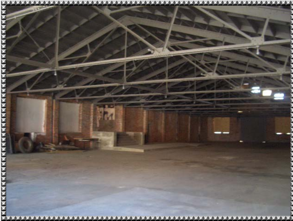
Clear Span Trusses
